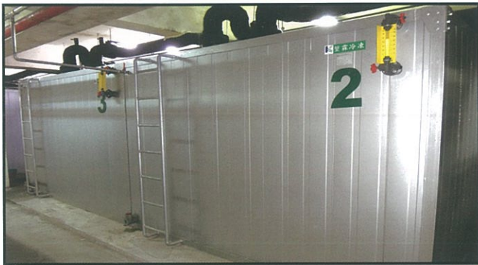
儲冰槽更新 Renewed Ice Storage Tanks
