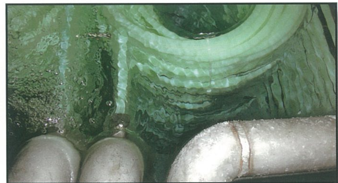
融冰冰水循環 Ice Melting with Chilled water Circulating
