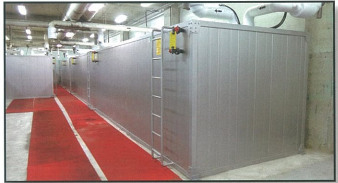
儲冰槽更新 Renewed Ice Storage Tanks
